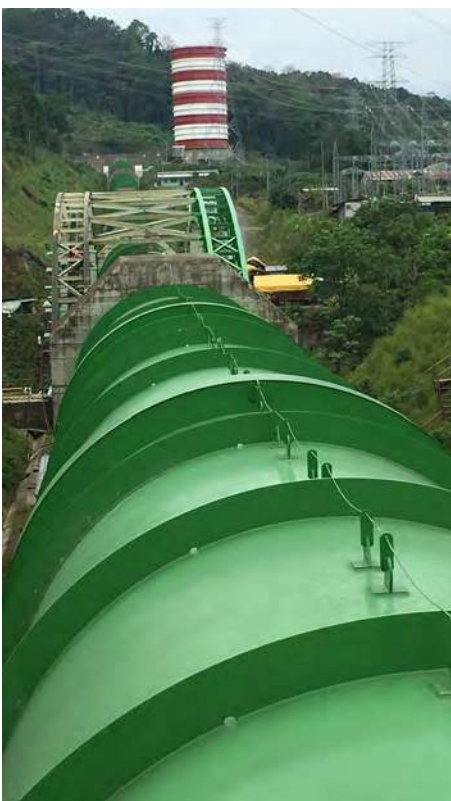
The powerhouse penstock and surge tower
